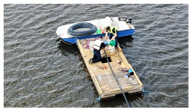
*Figure 3. Installation of the irrigation pump at the raft.*
